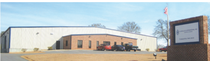
AIRCRAFT COMPONENTS AND GSE MRO FACILITY
